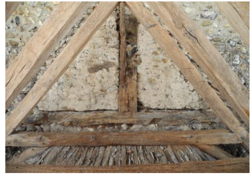
Truss 'fossilised' at the west end of the chancel roof
